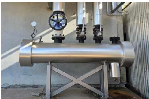
STEAM & CONDENSATE LINE SYSTEM FABRICATION
